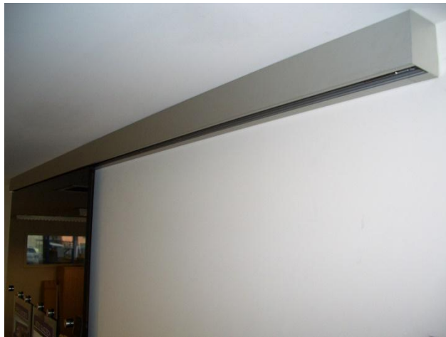
Figure 4: Typical GlassGlide top track.
