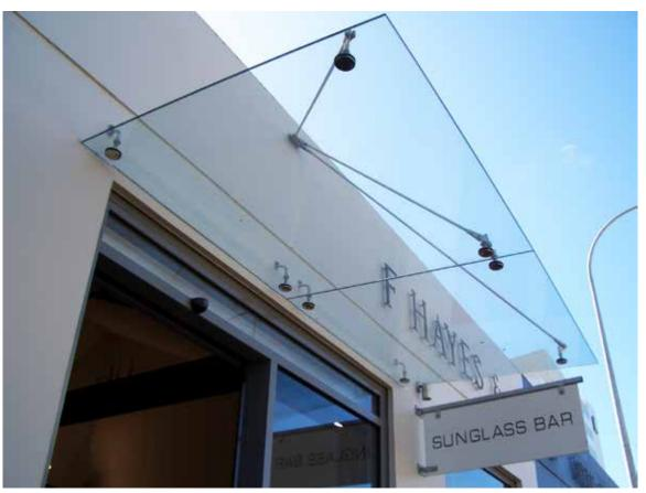
Specific Engineering design is required when tied back to a single fixing point.
