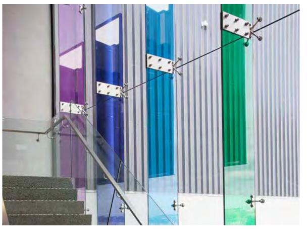
SAFELITE® EVA not suitable for splice plate assemblies shown in image above.
